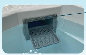
Once the filter housing has been removed, we now need to slide the filter tray.
