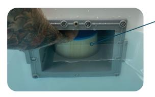
Lift the filter and remove the filter from its housing.
